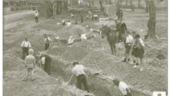
5 Jan. 1942, children watch on while local men dig slit trenches in Erskineville to give some shelter against a possible air raid attack from Japanese planes. The trenches were designed in a zig zag fashion in order to mitigate the blast effect of a direct hit (a design learnt in the early days of trench warfare during WWI). Many of these slit trenches were dug in the grounds of schools (including ours), shopping centres, local parks and were retained for the duration of WWII.
