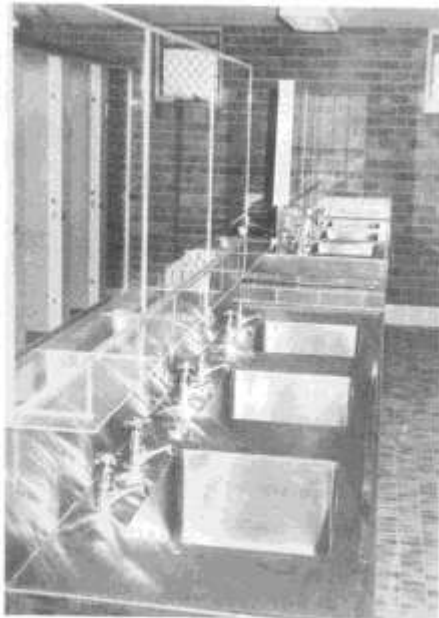
One of the bathrooms
