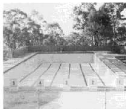
The newly painted pool
